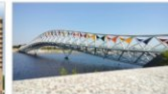
ATAL BRIDGE - AHMEDABAD
