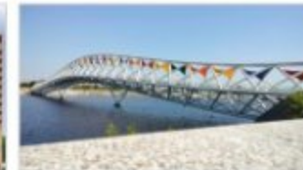
ATAL BRIDGE - AHMEDABAD
